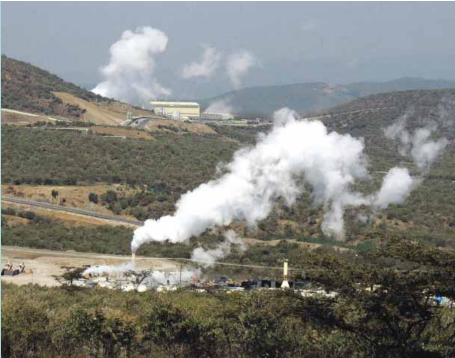
A geothermal power plant in Olkaria
