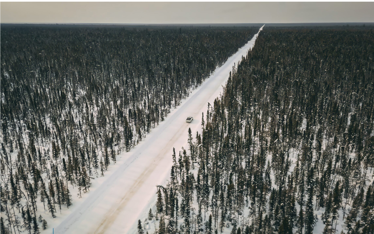
■ Winter road. Photo: Eleven North Visuals
